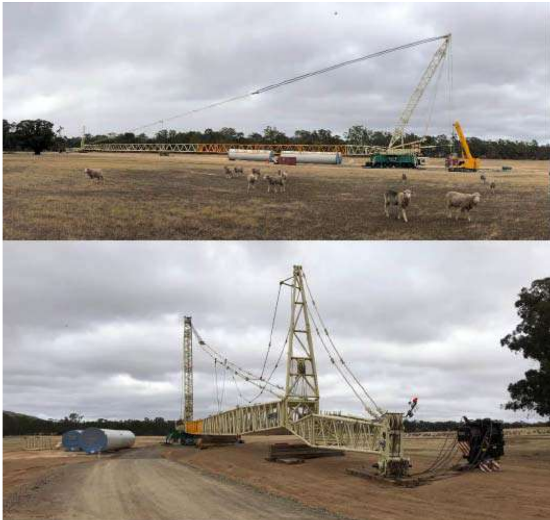
Figure 6 – Crane and Tower Sections
