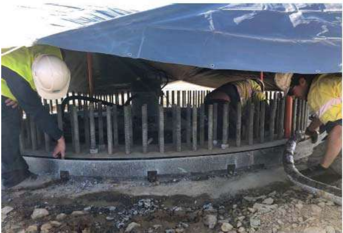
Figure 1 – Grouting Works Commenced
