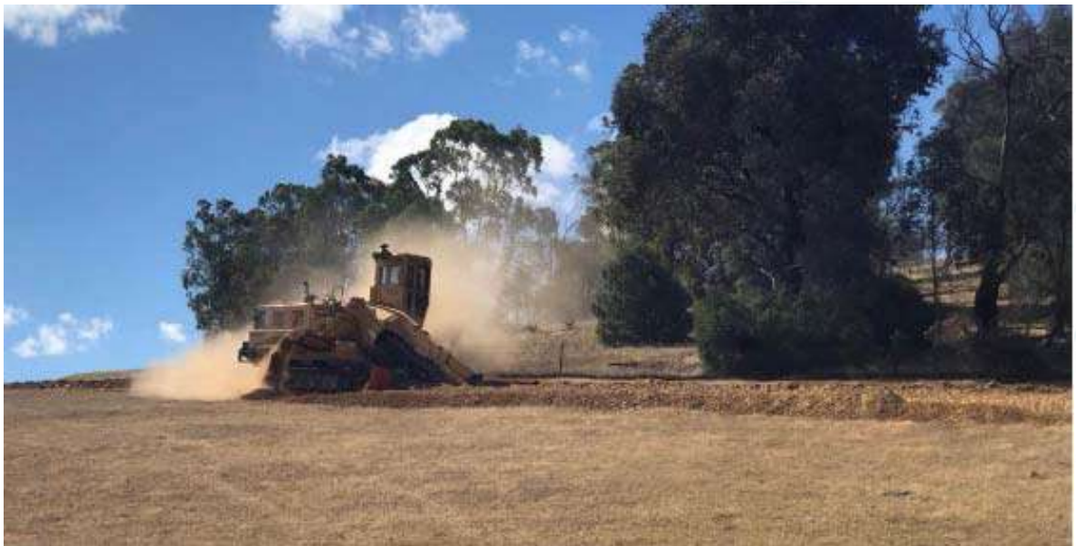
Figure 2 – U/G Cable Works
